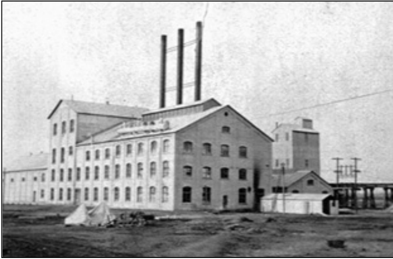
Newly-completed sugar factory in Layton. Layton Sugar Company began operations in 1915. The original officers were Jesse Knight, president; E. P. Ellison, first vice-president; David C. Eccles, second vice-president; James E. Ellison, manager. The initial investment was over one million dollars.
