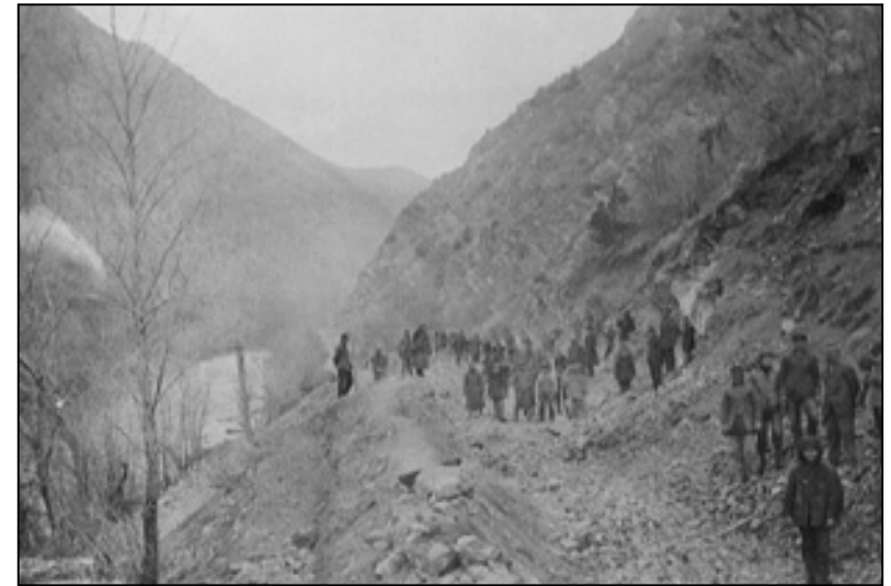
Building the canal system in Weber Canyon, 1881–82
