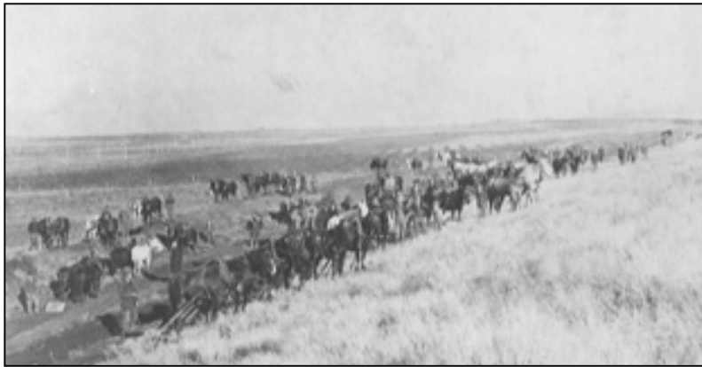
Extending the canal in the Roy area, 1910
