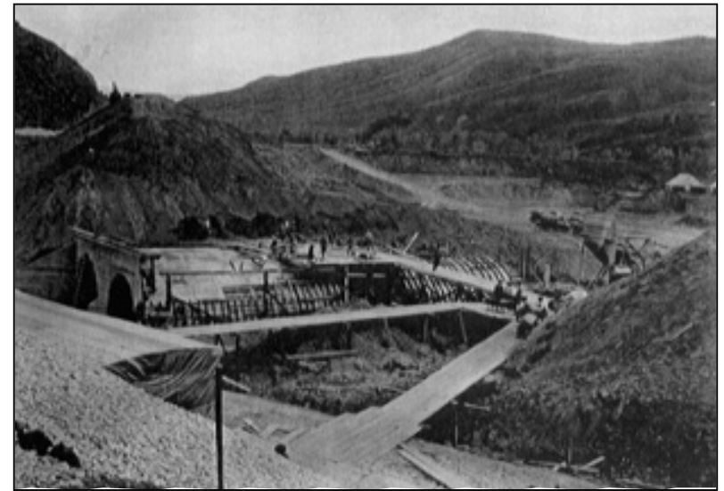
Echo Creek Arch Structure, ca. 1927 (Courtesy DWCCC Archives).
