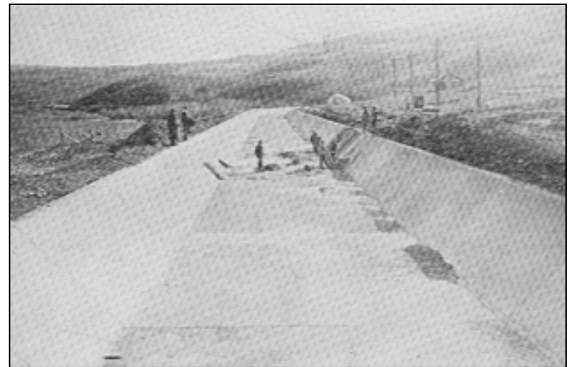
The company began lining its canals with concrete around 1910
