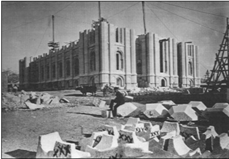
Hauling granite stones for the construction of the Salt Lake Temple
