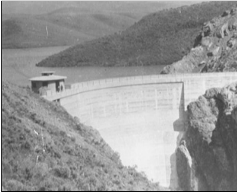
East Canyon Dam at its completion in 1915
