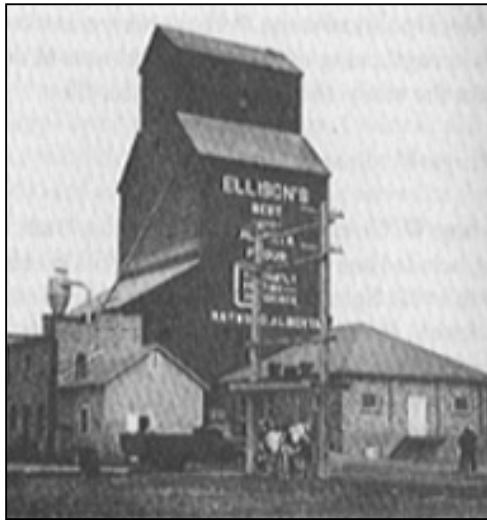
Ellison Mill and Elevator A at Raymond, Alberta. First built in 1902, burned and re-built twice, 1924–25 and 1937
